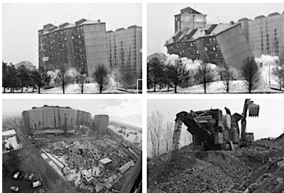
Fig. 3 Blast demolition and rubber recycling of the building (adopted from Blengini [61])
